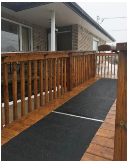
Figure 3.6 Ramp into Haley House
