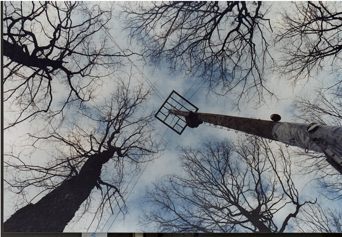
Plate 4. This photo is taken in March 2001, during the construction of the canopy access system. With the absence of vegetation the postman's walk and guy lines are clearly visible.
