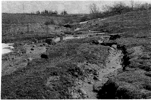
Photo 7: Washouts and bank erosion in April 1993. Notice the location of the large boulder in the stream.
